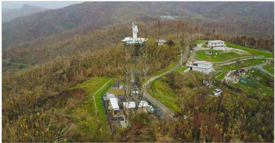
Figure 3.1-10. The remnants of the San Juan WSR-88D radar after its destruction by Hurricane Maria. Courtesy of WFO San Juan.
