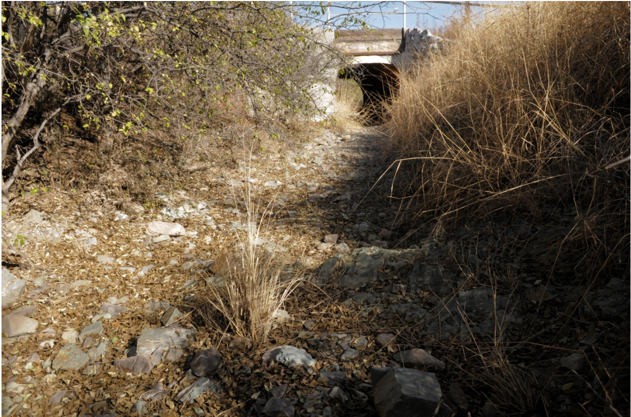
Figure 2. The dry wash and constructed bridge and culvert at Chilton Ranch.
